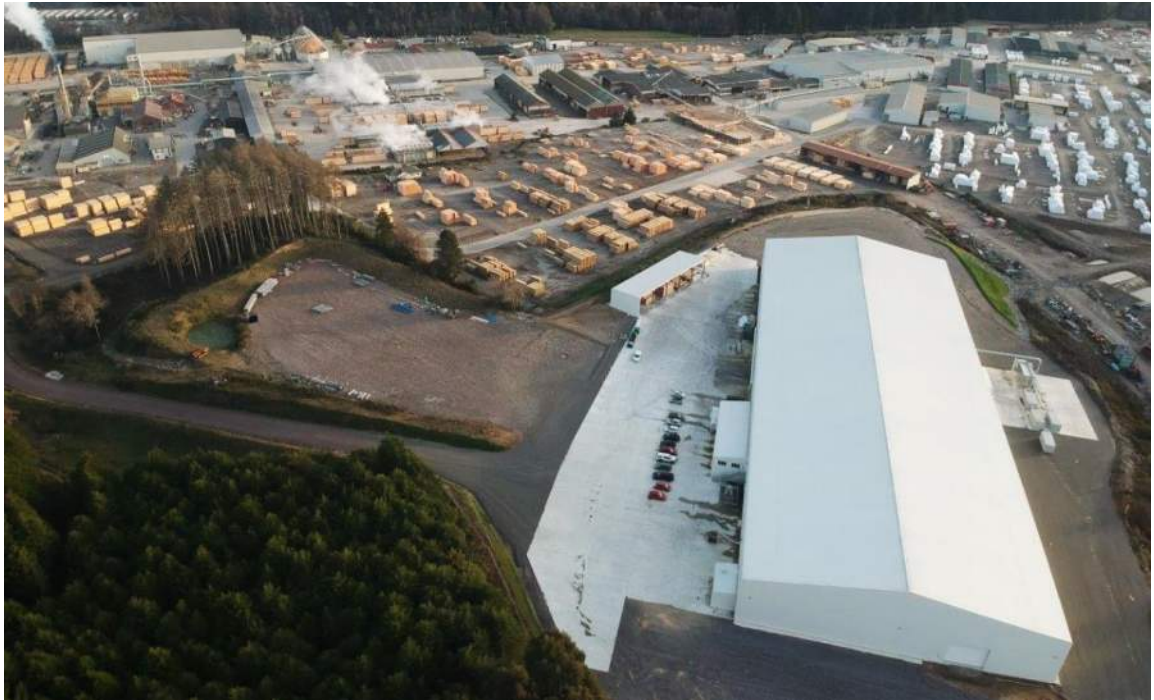
Figure 1: Red Stag's primary EWP site in Rotorua.
