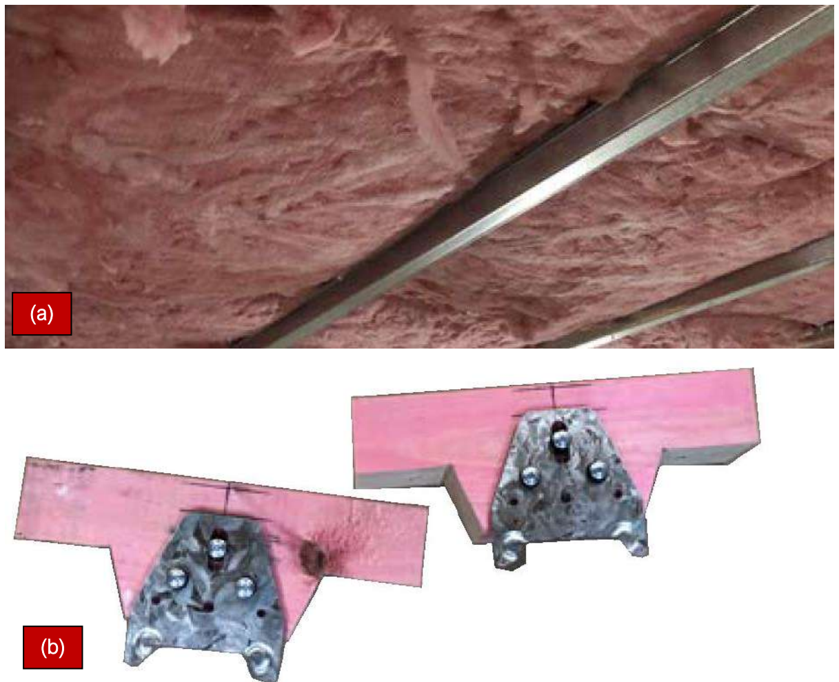
Figure 120: a) Rondo metal ceiling batten with thermal insulation; b) Gib quiet clip tying the metal ceiling batten to the underside of the flooring system.
