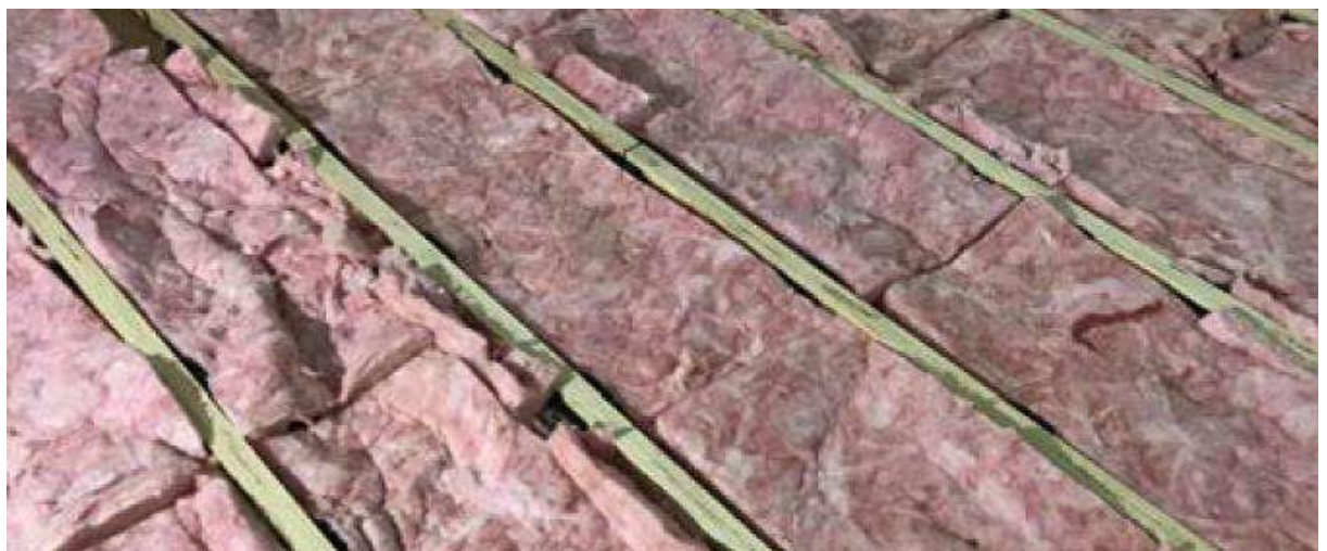
Figure 119: Cradle system with thermal insulation.
