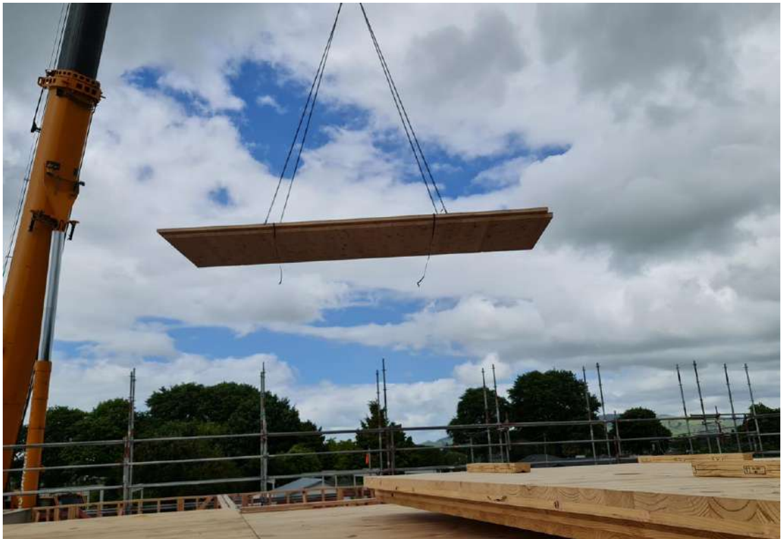
Figure 26: Example of four-point lifting solution for a 3 m x 8 m Red Stag CLT panel.
