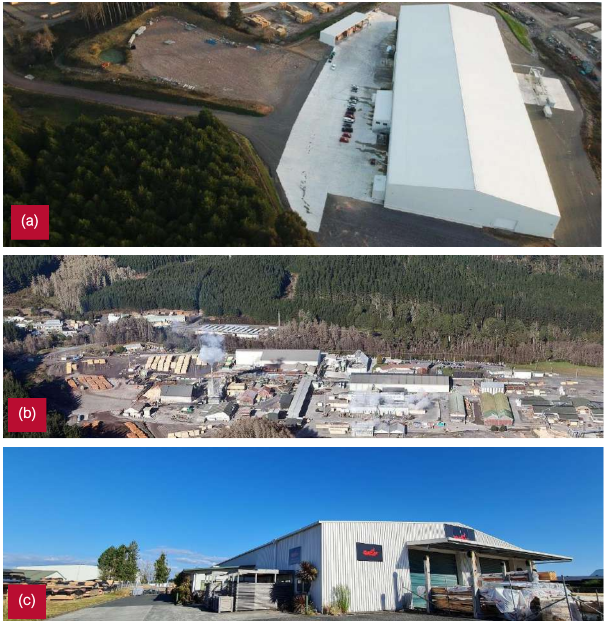
Figure 47: Red Stag Group of Companies; a) Red Stag primary EWP site in Rotorua, b) Red Stag Timber site in Rotorua, c) Red Stag Frame & Truss manufacturing plant in Hamilton.
