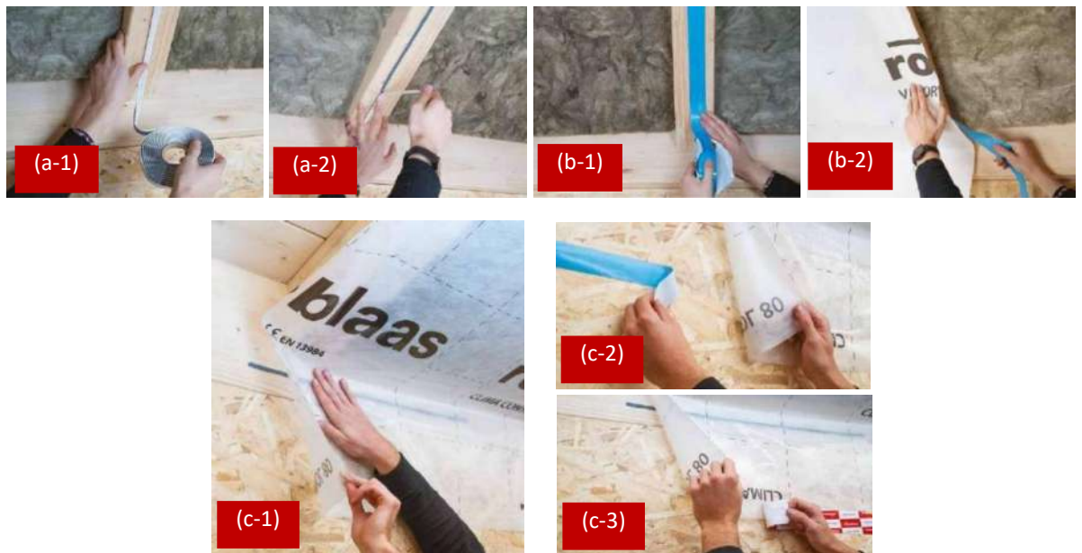
Figure 45: Application on internal side of the roof [14].
