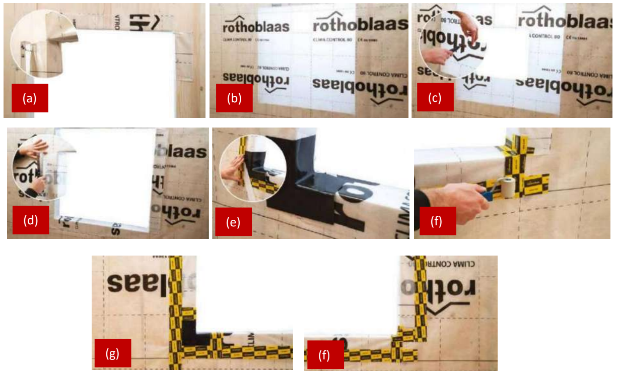
Figure 44: Membrane installation for wall penetrations [14].
