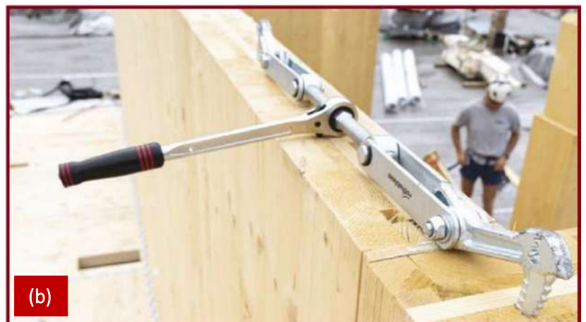
Figure 88: SKORPIO applications; a) SKORPIO utilised to pull CLT floor panels together; b) SKORPIO utilised to pull CLT wall panels together (pulling into a corner) [20] .
