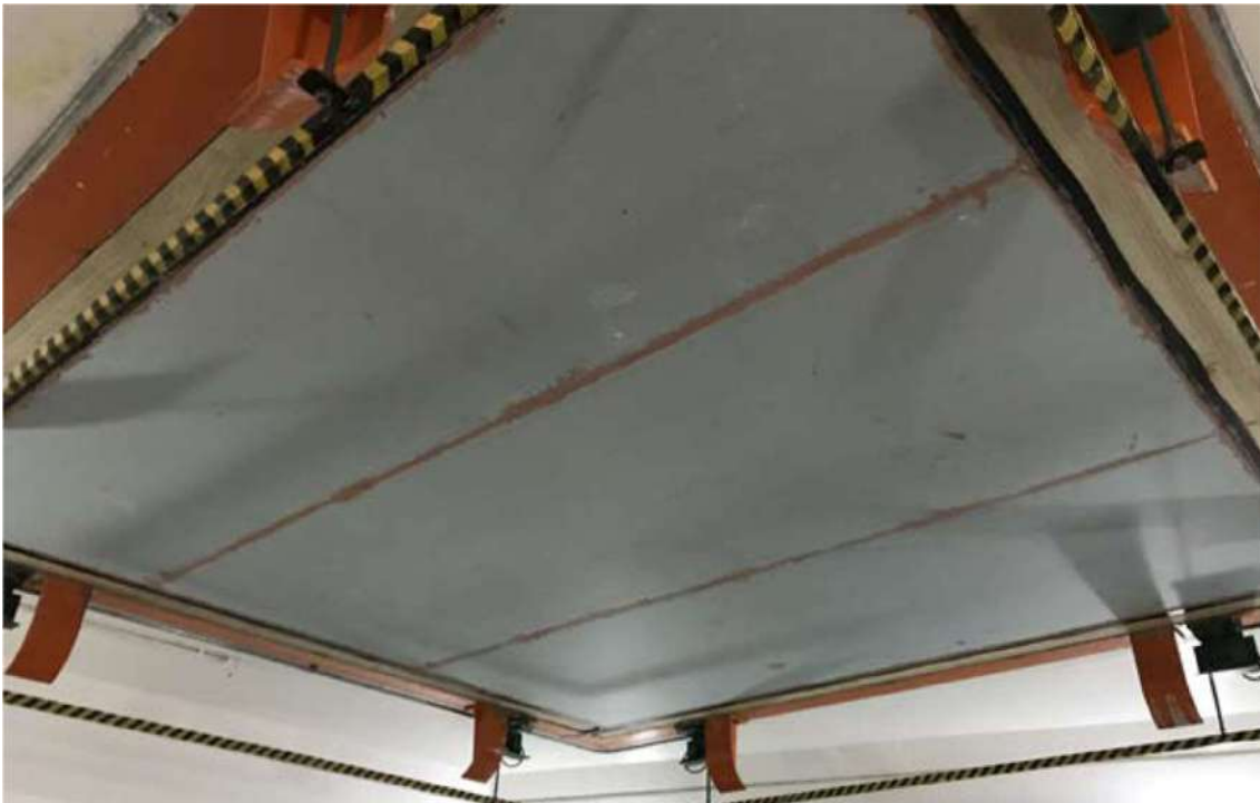
Figure 135: Suspended ceiling in the lower chamber.
