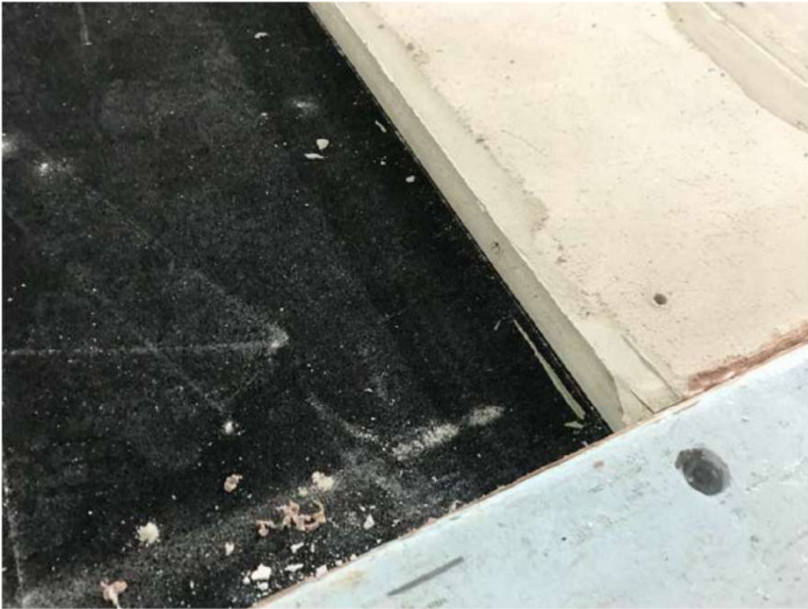
Figure 134: Underlay and upper layer installation.
