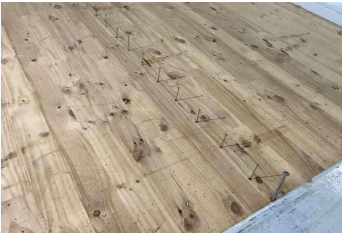
Figure 133: Three-layer Red Stag CLT panel with lap joint.
