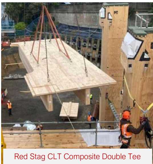
Figure 158: Red Stag CLT composite product installation in Living Pa Project site, Wellington/New Zealand.
