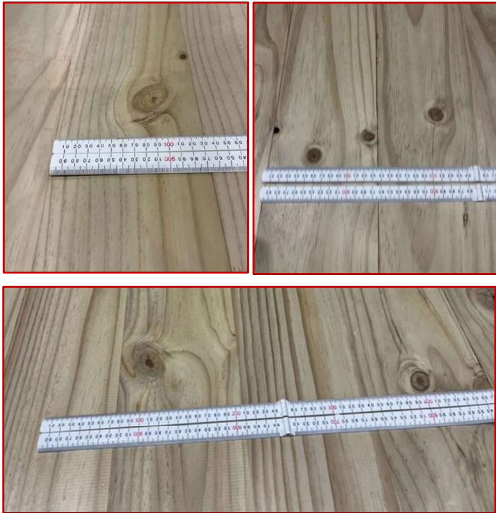
Figure 142g illustrate common grading inclusions in standard grade EWP. Represented dimensions in the figures are examples only and should be considered in addition to the details provided in section 50.1 above.
