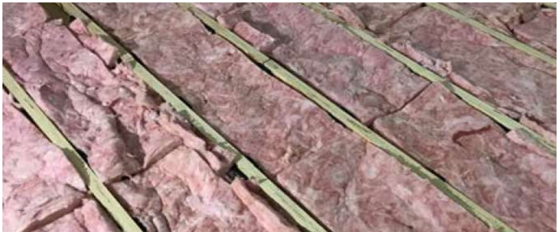
Figure 129: Cradle system with thermal insulation.
