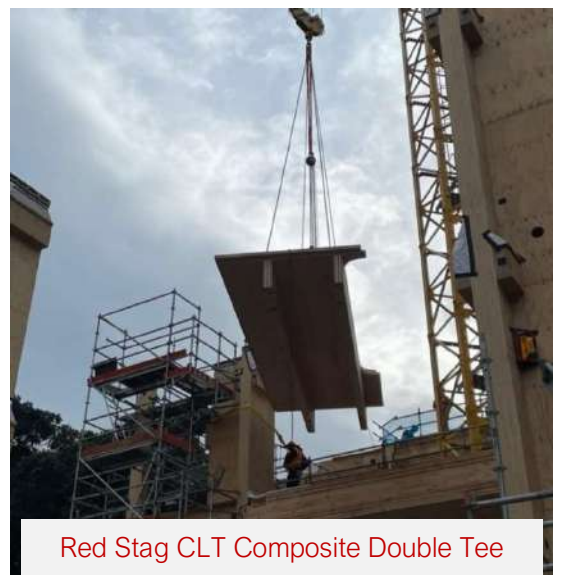
Figure 158: Red Stag CLT composite product installation in Living Pa Project site, Wellington/New Zealand.
