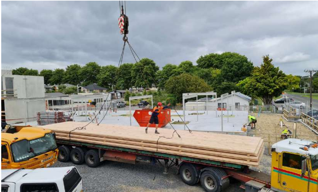
Figure 27: Site safety officer is checking all equipment and components related to the lifting process.
