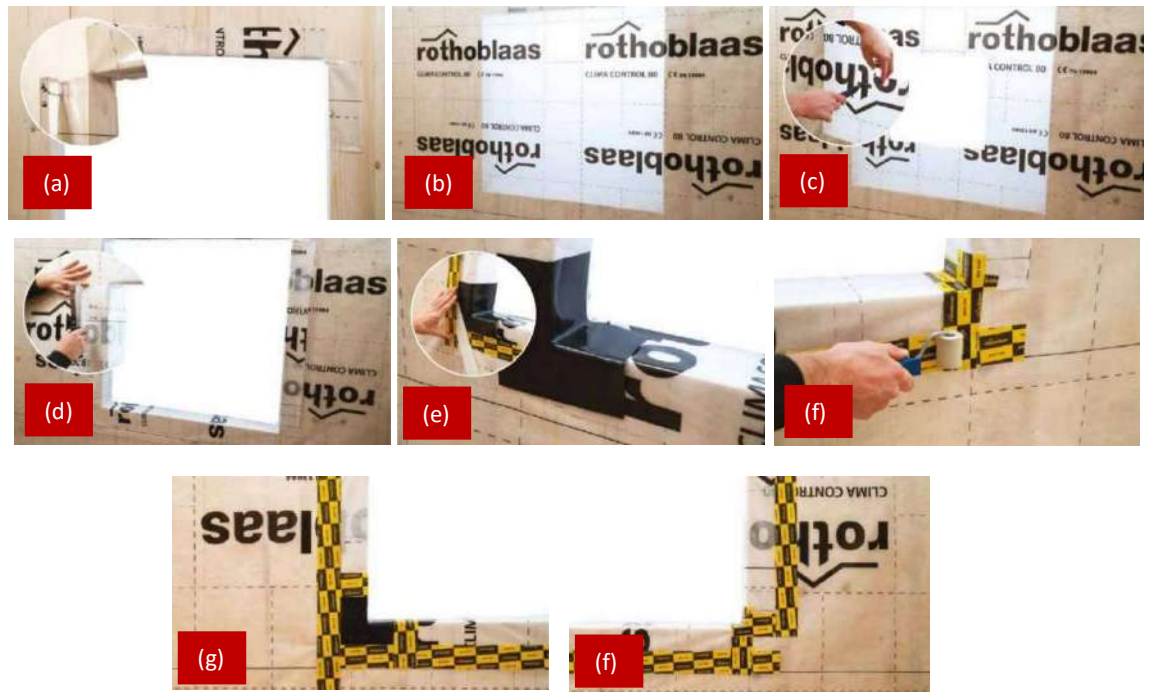
Figure 44: Membrane installation for wall penetrations [14] .
