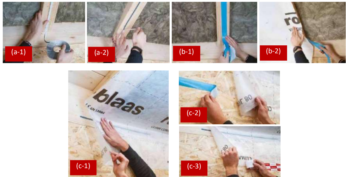
Figure 45: Application on internal side of the roof [14] .
